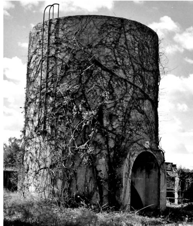
Sand storage silo
